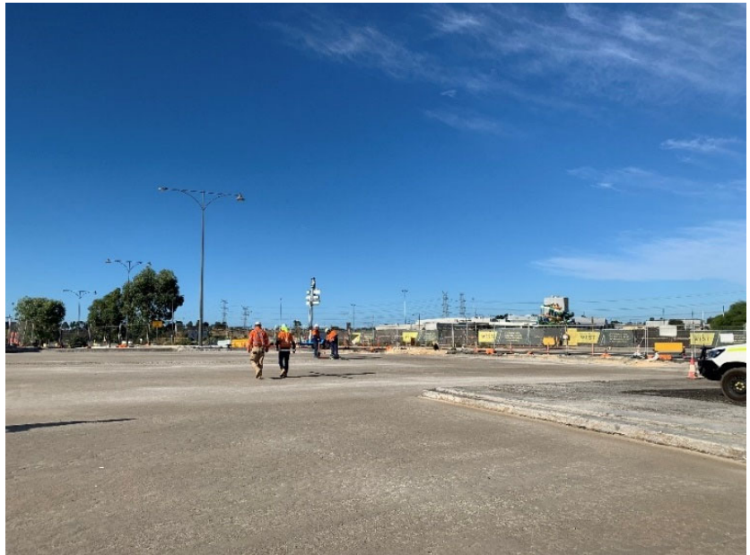
Crushed Recycled Concrete trimmed and compacted at the North Lake Road Intersection
