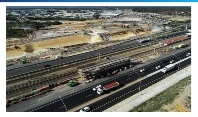
Less than eight months into construction, the project has achieved a significant milestone with completion of excavation and concrete works at its central bridge pier on Kwinana Freeway. This is the first critical step in connecting Armadale Road and North Lake Road over Kwinana Freeway.
