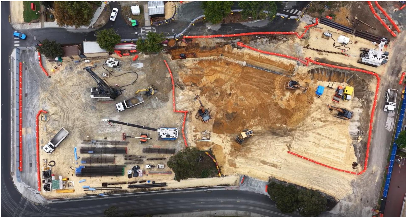
Aerial view of piling activity
